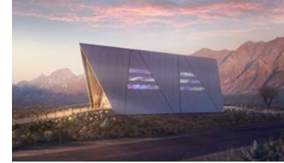
Oklo (shown) Approximately a dozen in development
